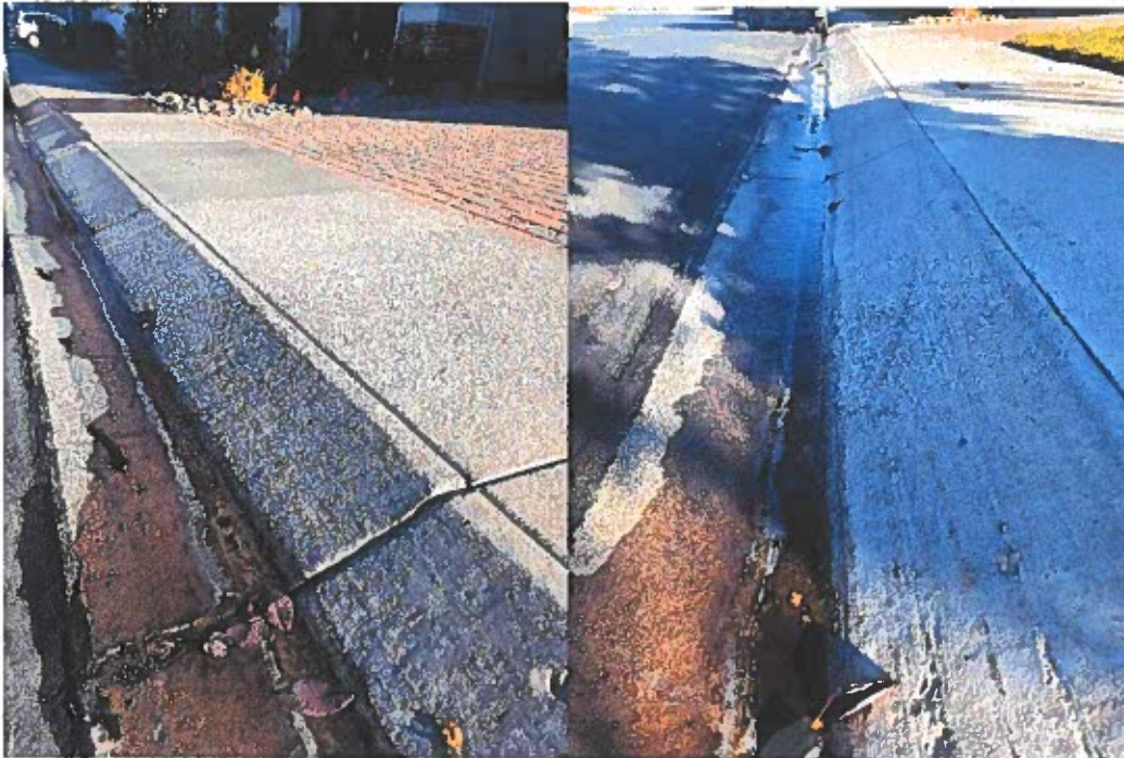
CRACKS ARE APPEARING AND THE SIDEWALK IS SINKING AND CRACKING DUE TO THE CONSTANT WATER FLOW.
