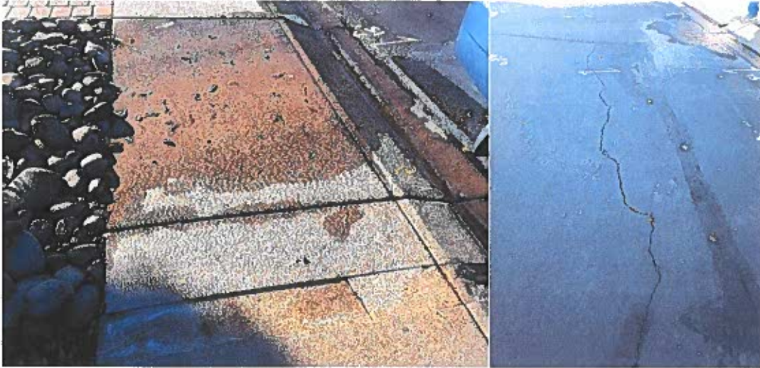
CRACKS ARE APPEARING AND THE SIDEWALK IS SINKING AND CRACKING DUE TO THE CONSTANT WATER FLOW.
